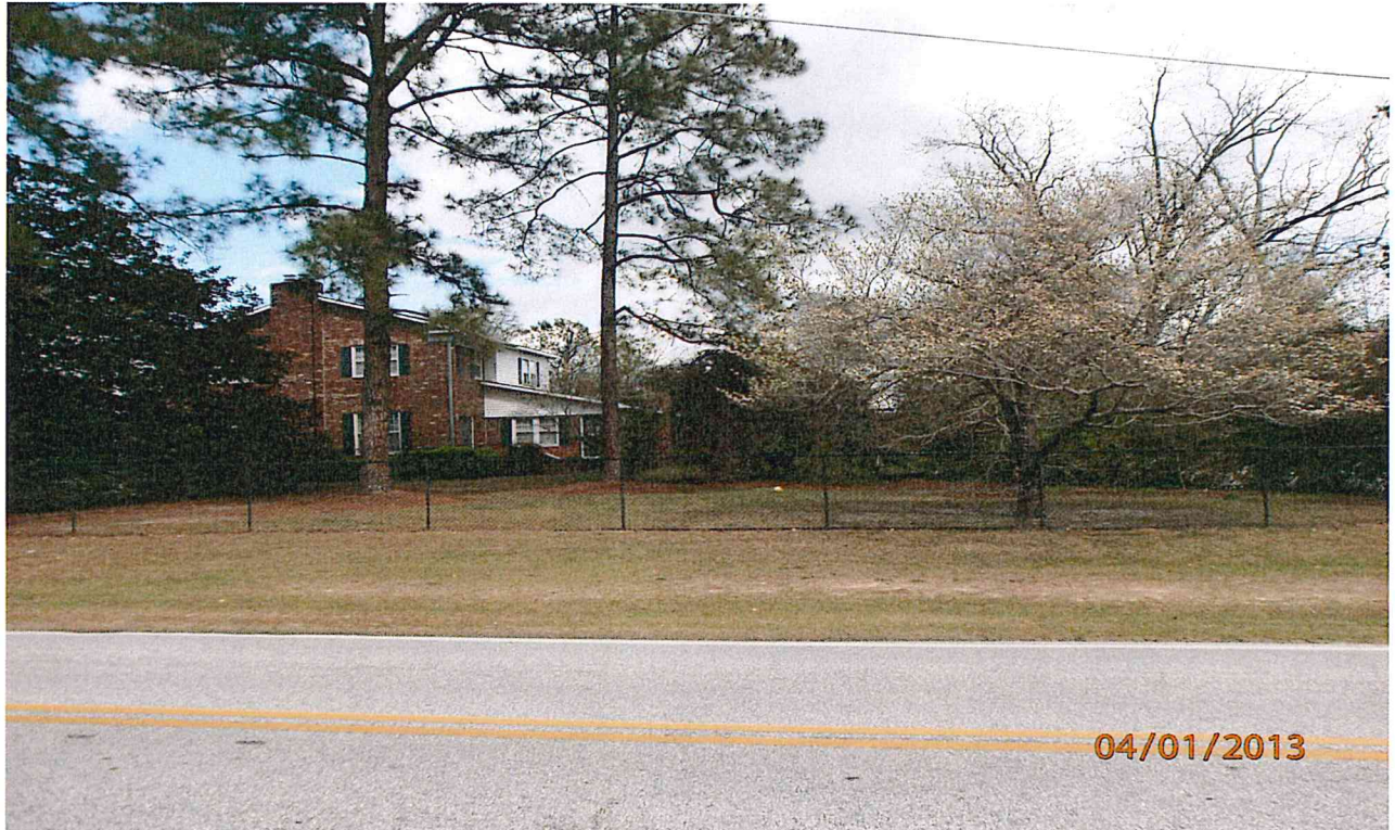
Figure 2: Vacant Single Family Home located across Cawana from Subject Site (also being considered in AN 13-04-05 for R4 Zoning).
