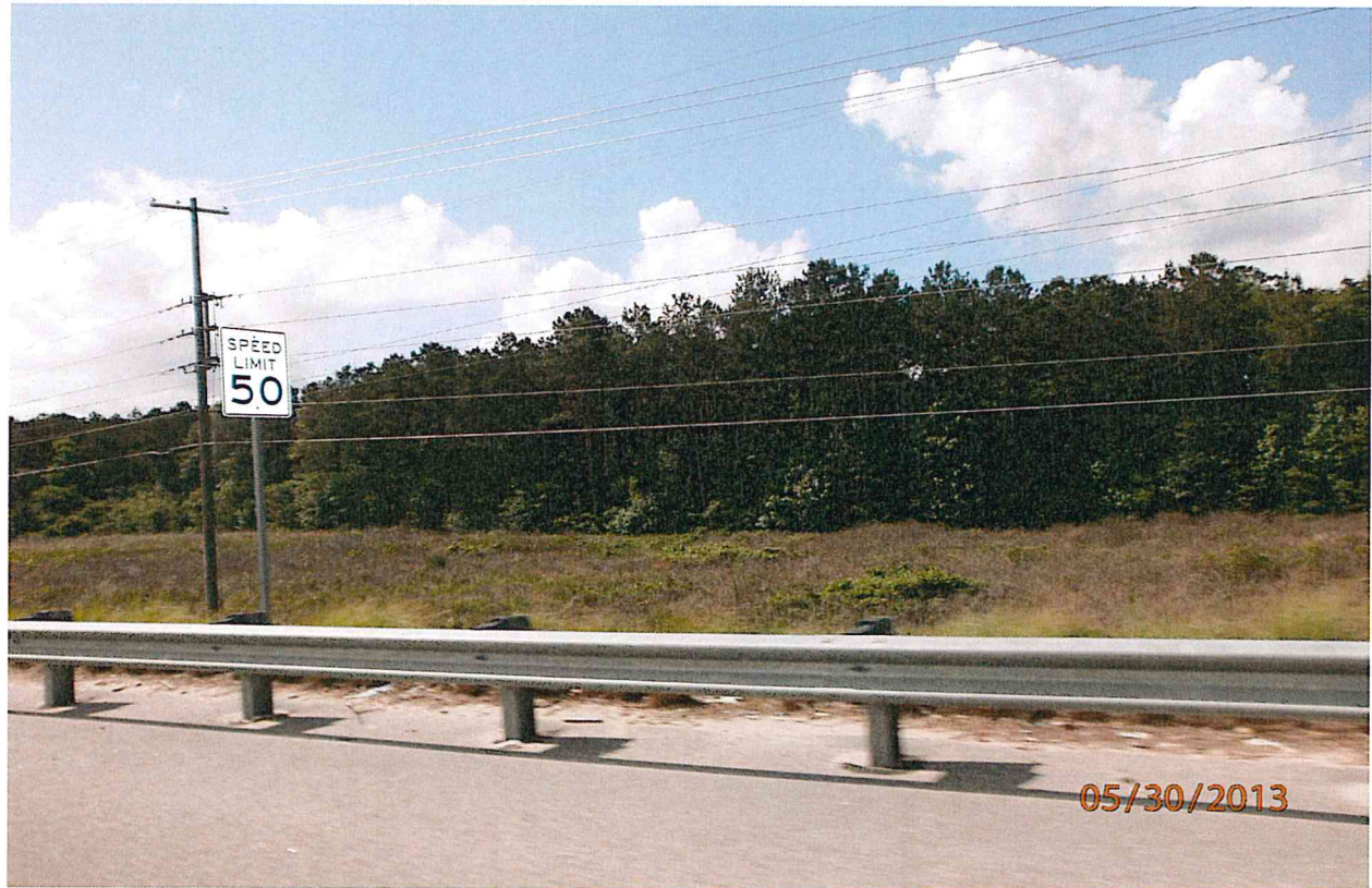
Figure 1: Subject Property from Veterans Memorial Parkway.
