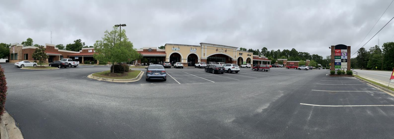
Picture 2: Looking northeast from the subject site, currently a commercial shopping center.
