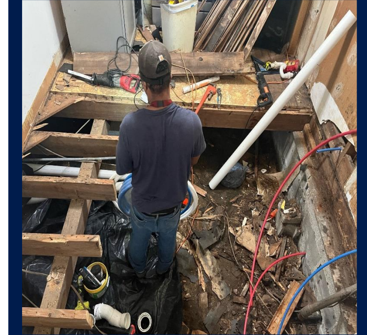
Damaged Subfloor
