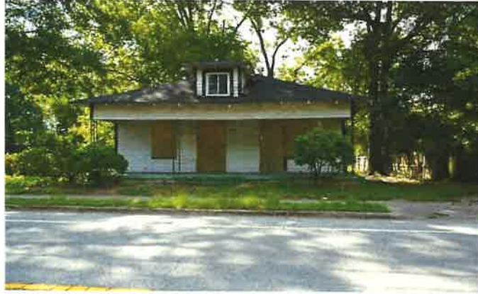
Vacant Homes on Johnson Street (above/below)
